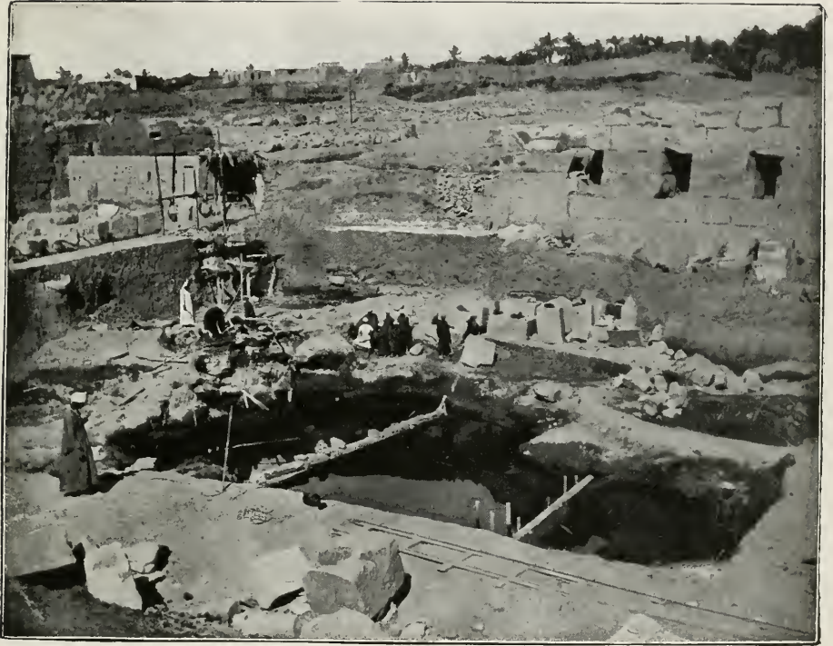
THE WORKS AT KARNAK IN JANUARY, 1906.
